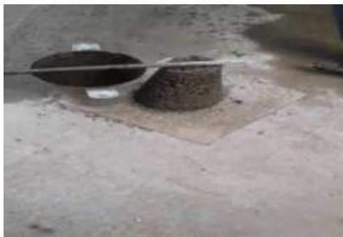
Fig. 7. Slump test of the concrete
