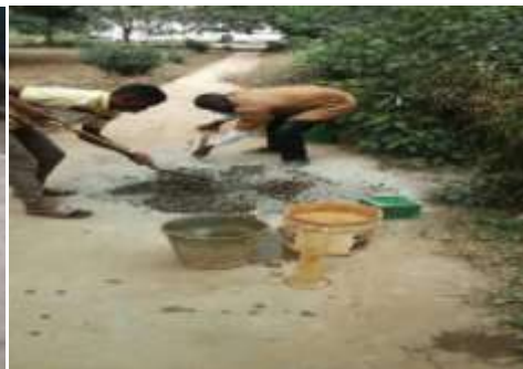
Fig. 8. Mixing of concrete
