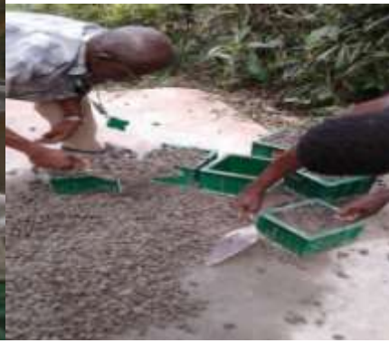
Fig. 4. Placing the mixed concrete into the Moulds
